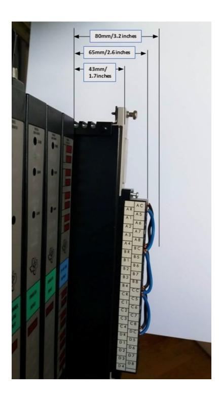
Note: The above dimensions are close approximations. When preparing for the installation use these dimensions to determine the clearances required inside the control cabinet which houses the existing 500 Base.
